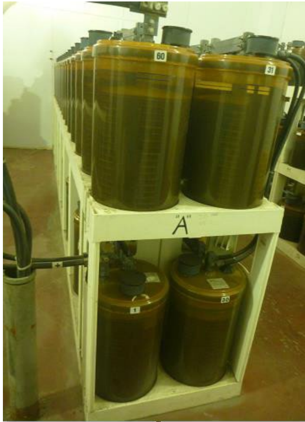
Station Service A – 60 1600AH ATT Round Cells – Center of Room.
